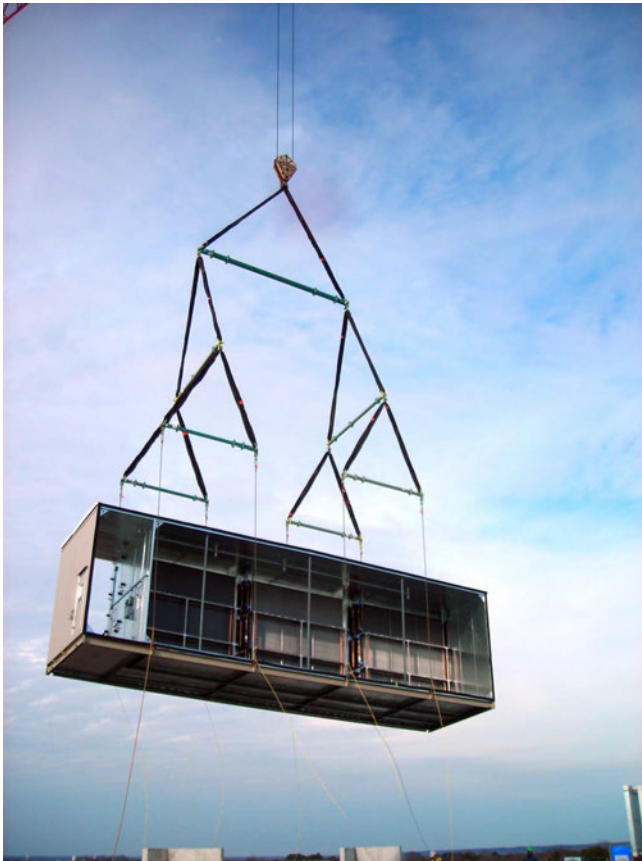
Figure 3. Use proper lifting and rigging methods
