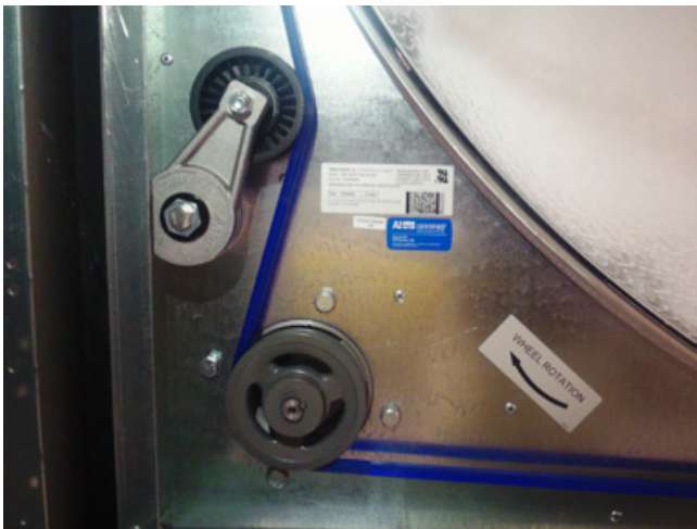
Figure 68. Confirm proper belt tracking on the wheel rim
